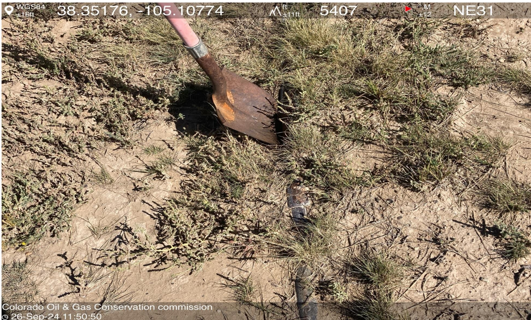
PHOTO 7: 2" FLOWLINE FOUND APP. 30 YARDS EAST OF LOCATION RUNNING TOWARD THE AREA WHERE THE HOUSE USED TO BE.
