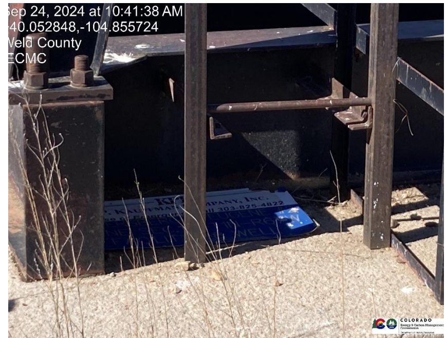
Pic 2 wellhead sign needs to be hung back up where visible
