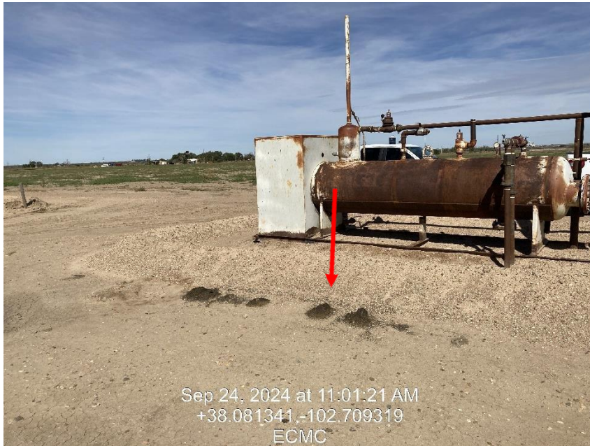
Photo 9 – Impacted materials observed near Heater Treater
