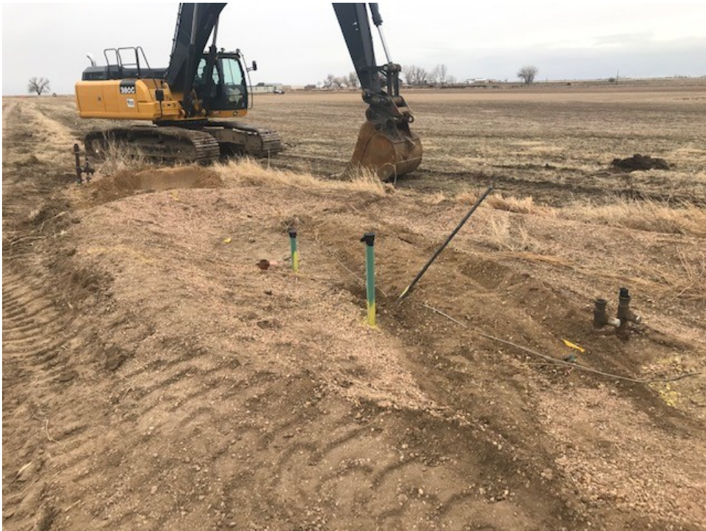
#4 – Former Separator Location
