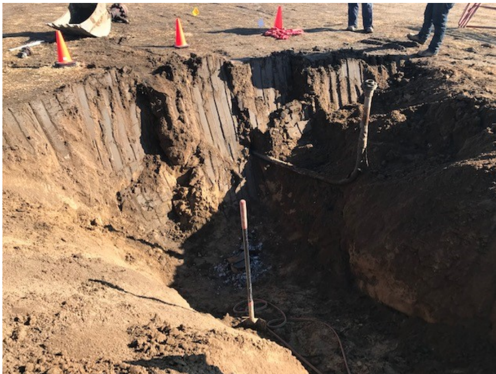
#6 – Looking Northeast at Wellhead Cut and Cap Excavation
