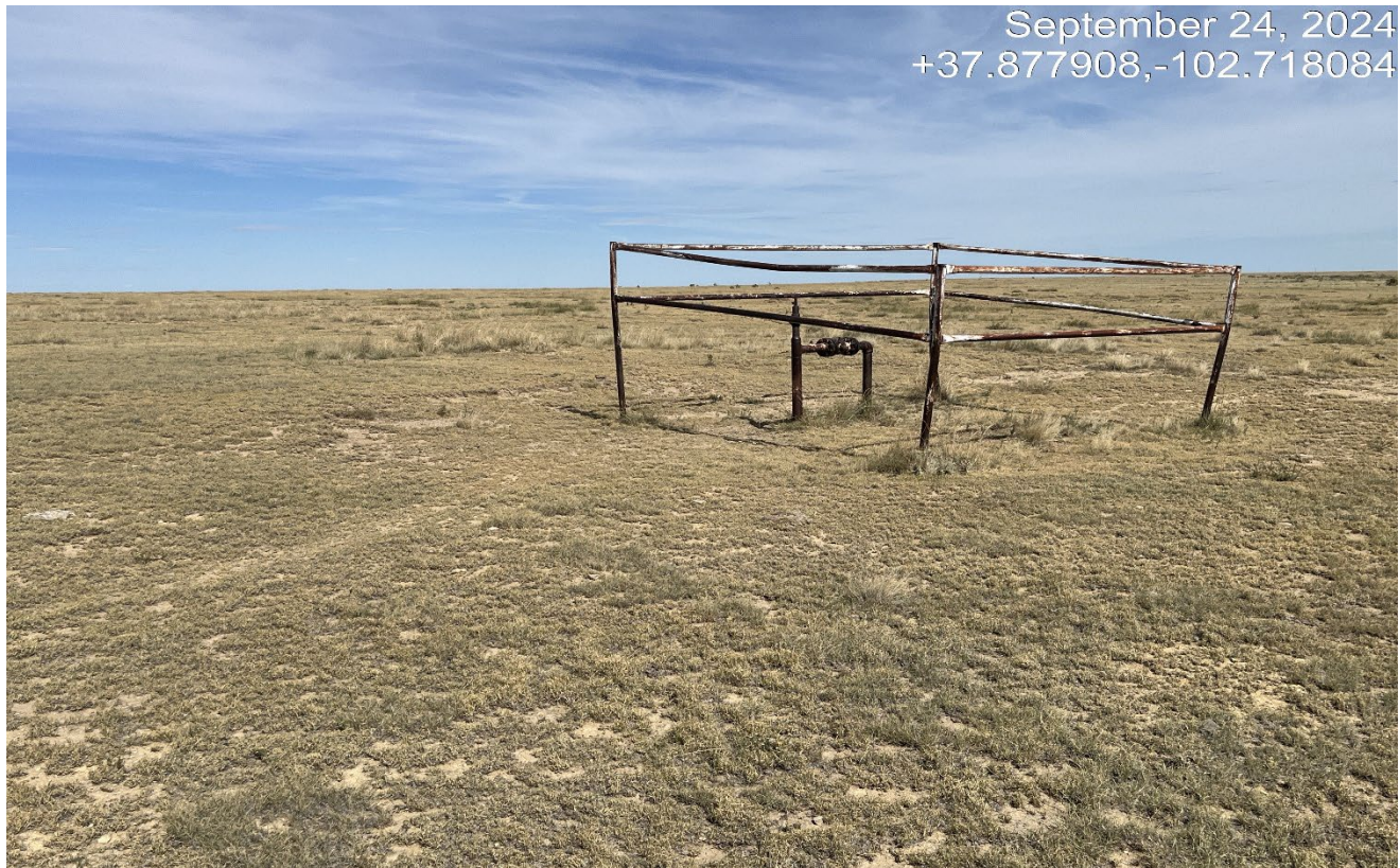
Photo 5. Another pipe riser associated with the well site was found at Lat/Long:37.87789,-102.71800. All equipment/risers need to be removed.
