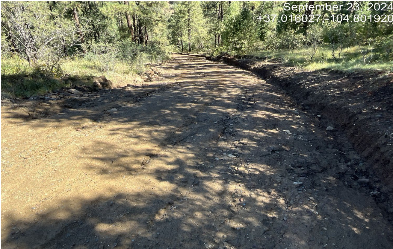
Photo 2. Facing back down the road at the wellsite. The road has been graded but no stormwater controls were installed. E.G. gravel, check dams, ect.
