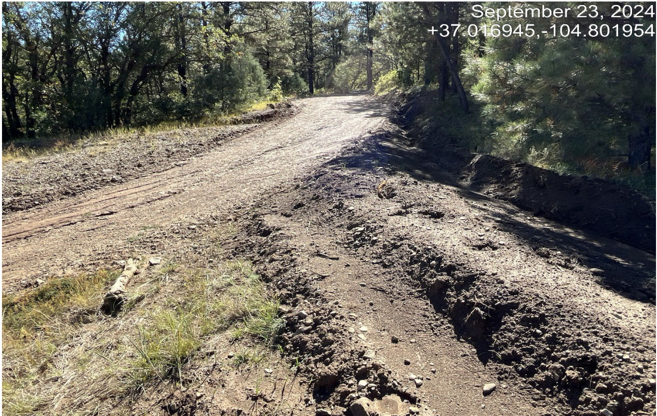
Photo 1. Facing south along the access road. This stormwater diversion was cleaned out. The disturbed soils need to be seeded for stabilization.
