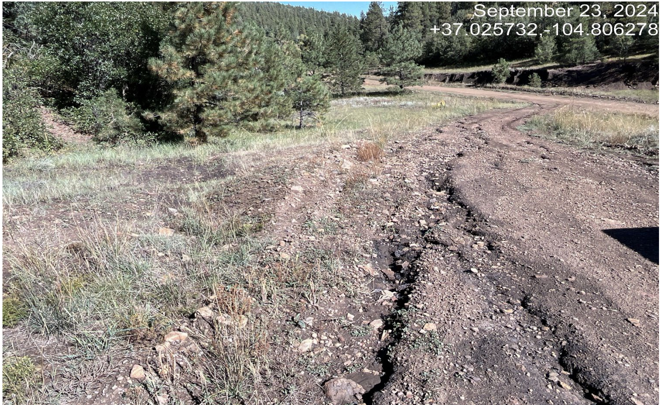
Photo 3. Facing north toward the access road. Stormwater needs to be diverted off the road.
