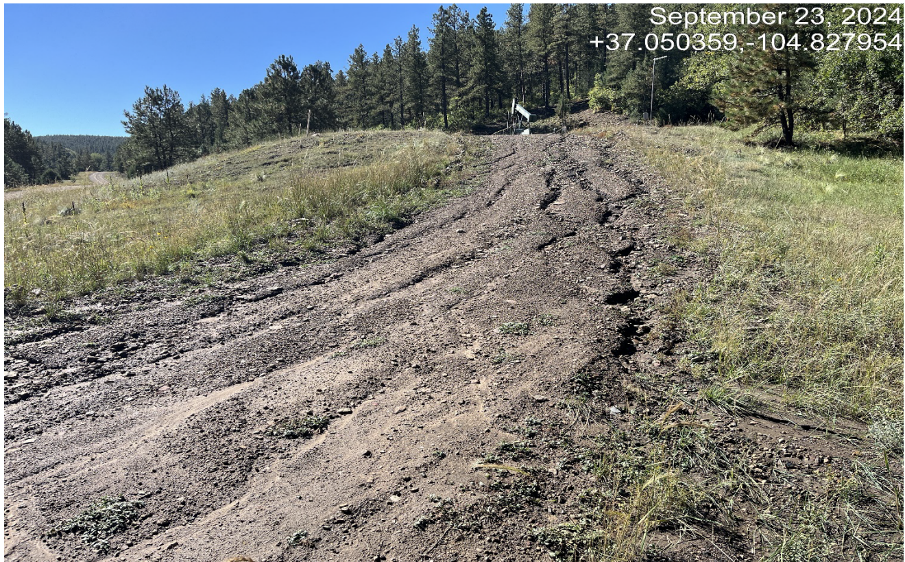
Photo 1. Facing southwest toward the access road where erosion is occurring.
