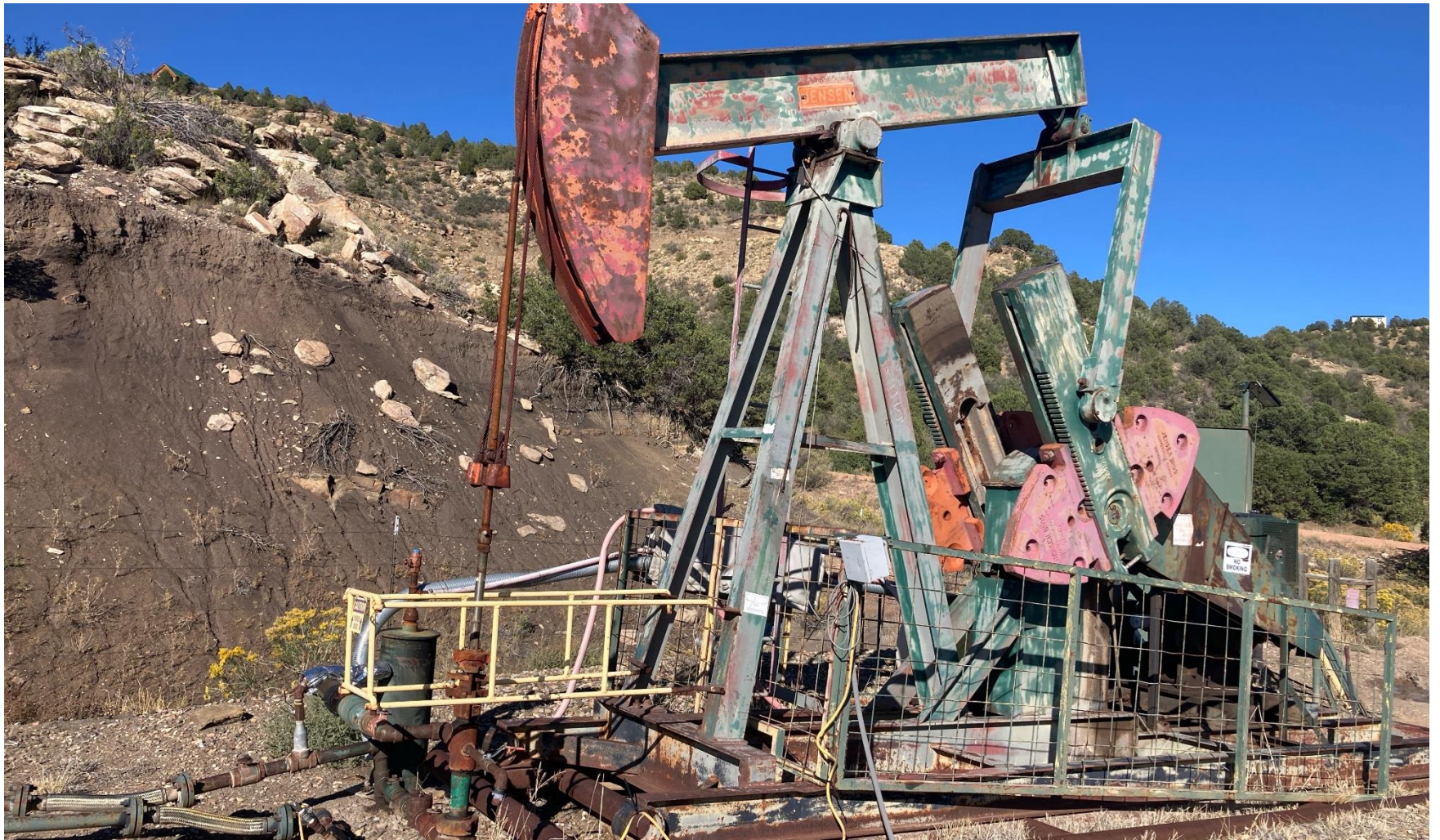
PHOTO 3: WELLHEAD AND EQUIPMENT
