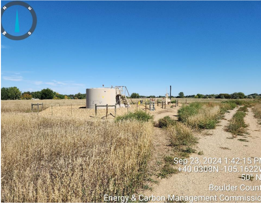
Photo 3 tank battery, production equipment
