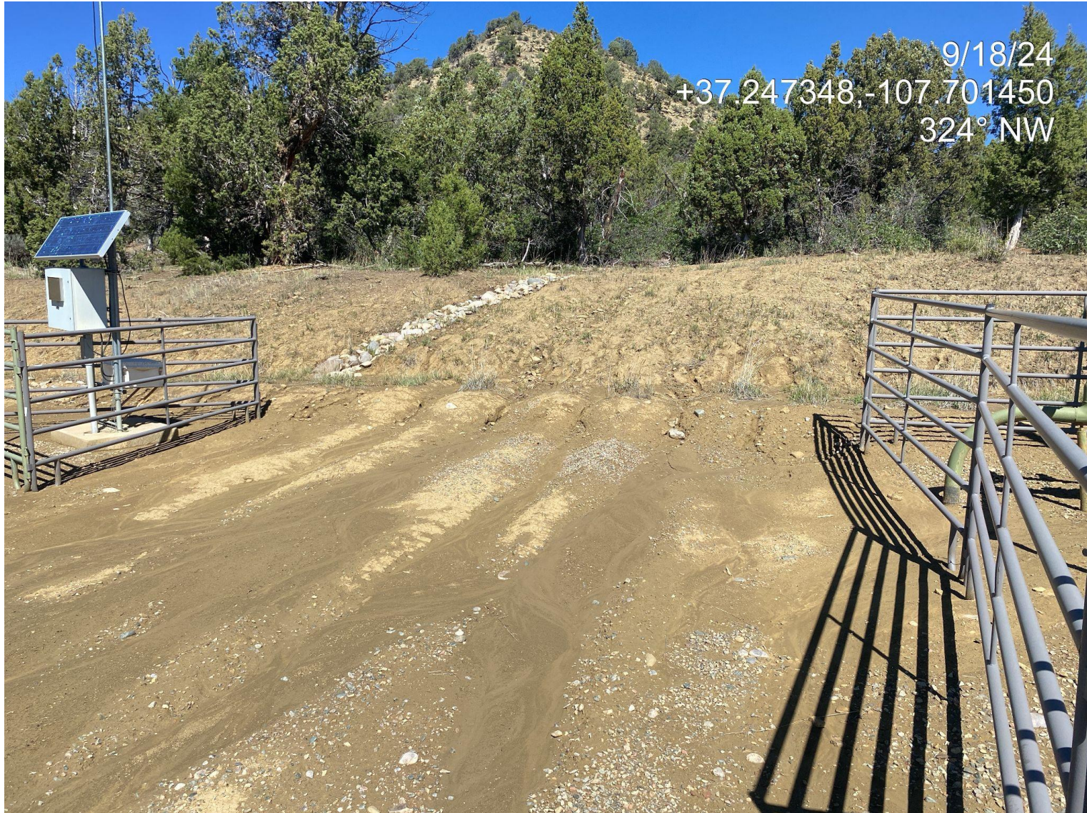
Photo 2. View of active erosion and sediment transport occurring on the northern edge of the active pad. Stormwater BMPs are needed in this area.
