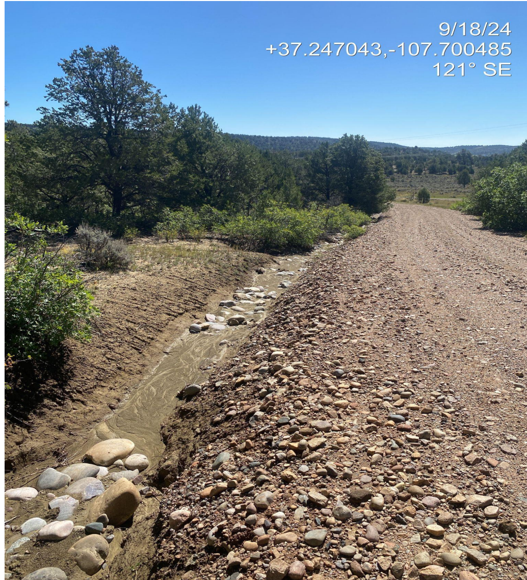
Photo 3. View of check dams along access road that are filled with sediment and no longer functioning.
