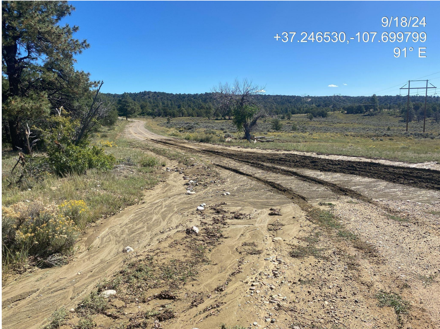
Photo 4. View of severe sediment deposition occurring at the location access point, as deep as a 10 inches in some areas.
