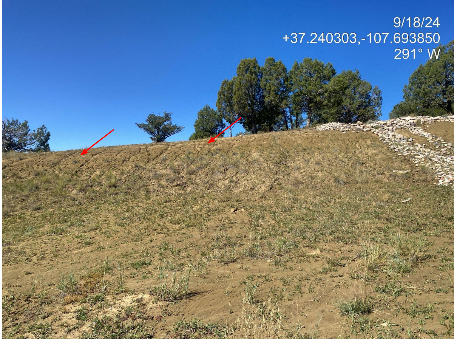
Photo 2. View of rill erosion issues persisting in the western portion of the disturbance, stormwater BMPs/additional stabilization are needed in this area.
