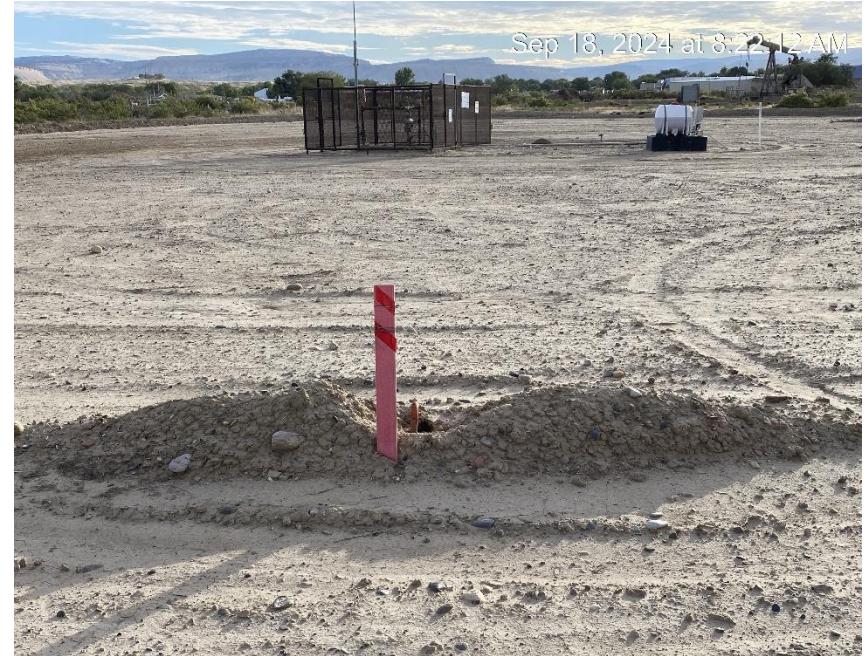
Location from Southwest corner
