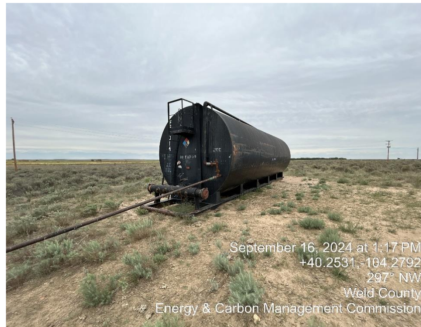
Tank needs secondary containment
