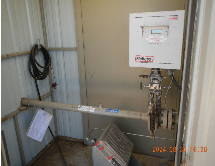
3. Gas meter inside meter shed.
