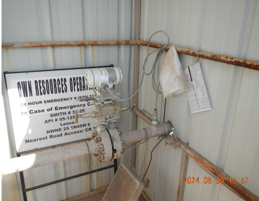
5. Gas meter inside remote gas meter shed.
