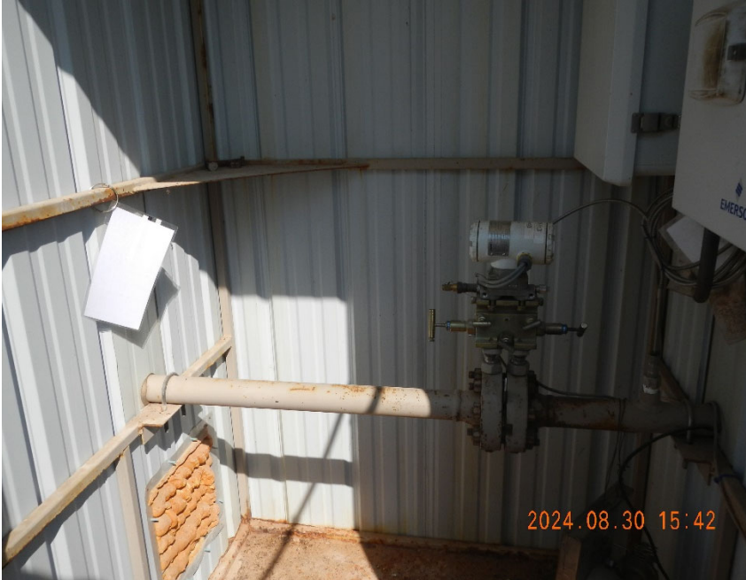
5. Gas meter inside remote meter shed.
