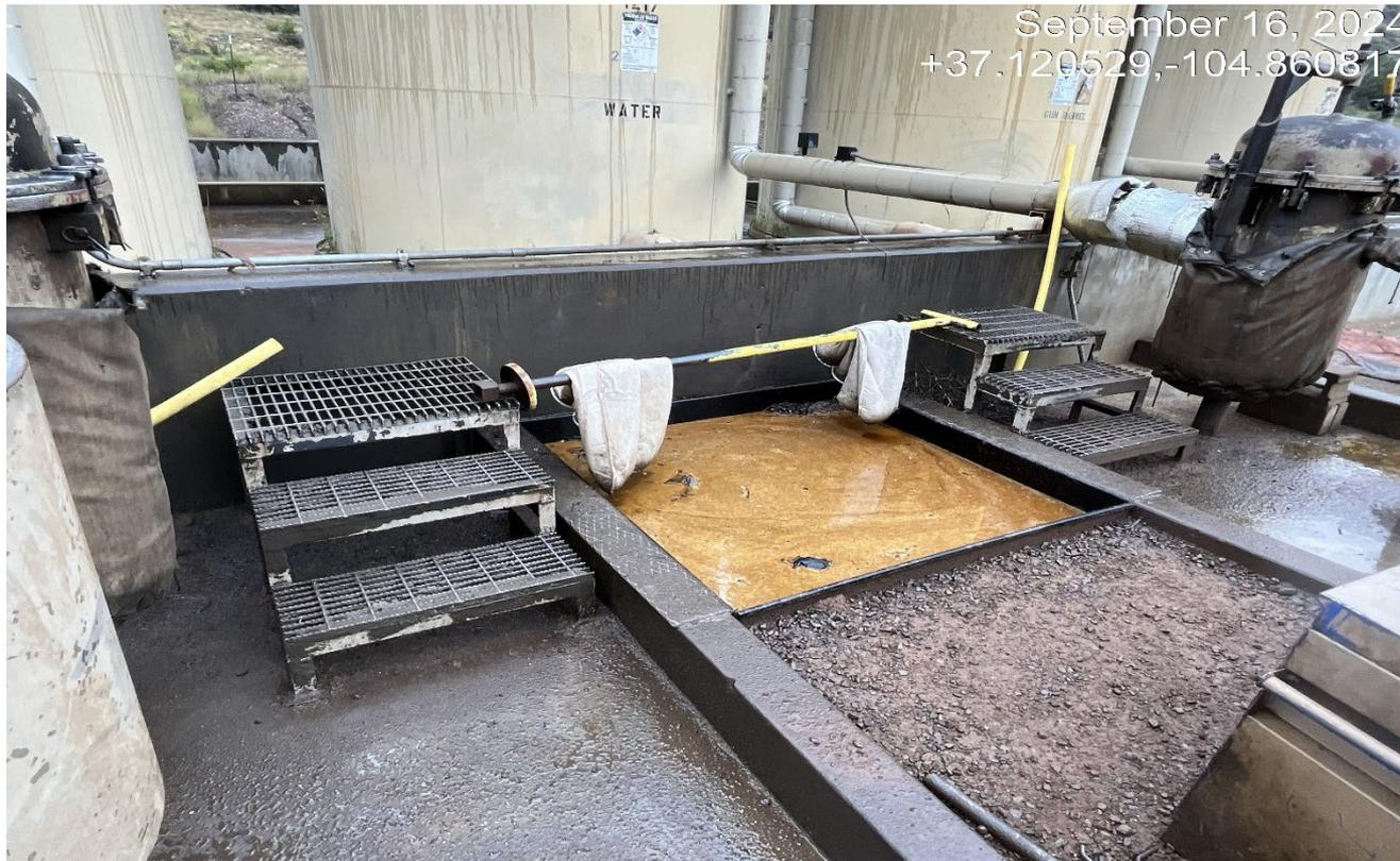
**Photo 6.** There is oily fluids in the secondary containment. Additionally netting must be installed to prevent wildlife entry. Previous CA was not completed.
