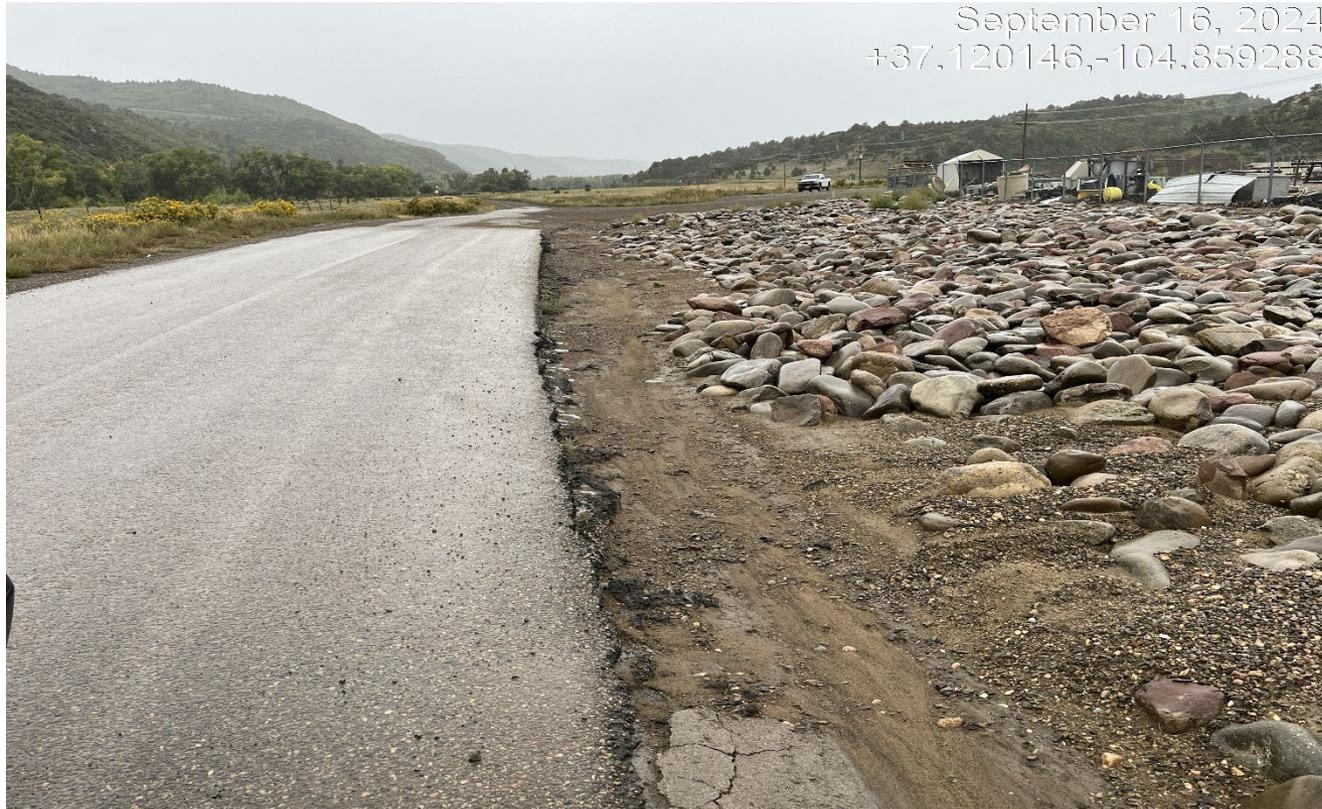
**Photo 1.** Facing southwest along the main road to the production facility. The sediment along the roadside has been cleaned out to allow storwater drainage to the culvert.
