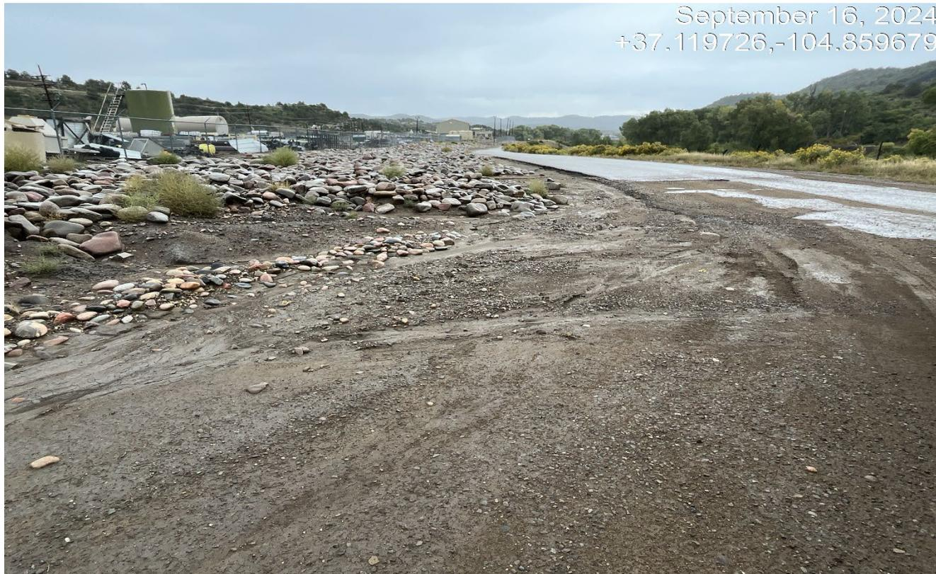
**Photo 3.** Facing back toward the main public road. Sediment needs to be cleaned off the road and vehicle tracking controls need to be implemented.
