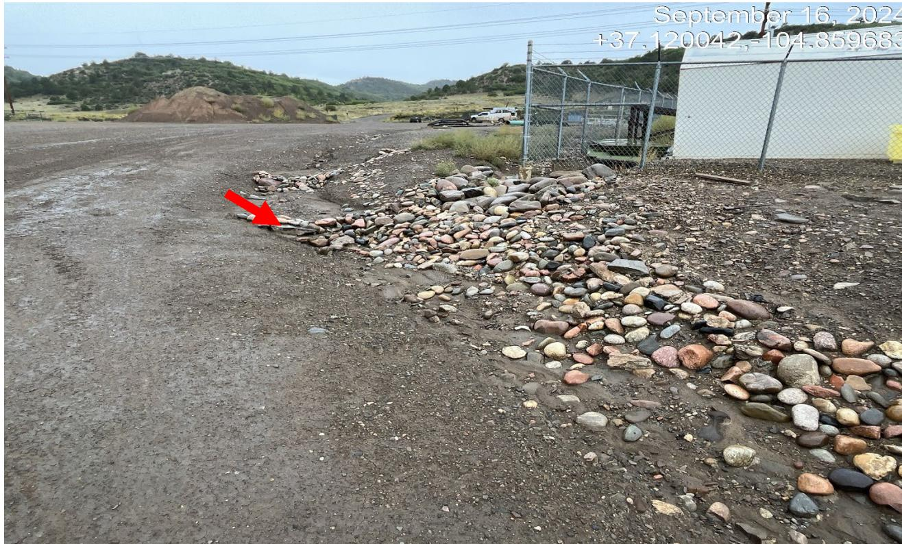
**Photo 2.** Facing west at the road to the production facility. There are rock check dams that have already filled in with sediment and need to be cleaned out. A larger sediment catch may be better to prevent sediment transport onto the road. Also, round rock does not lock together and can easily be displaced.
