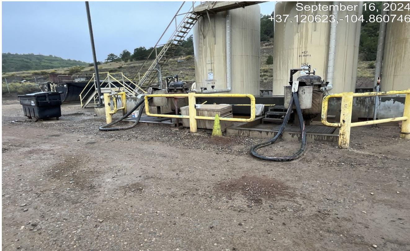
**Photo 7.** Facing toward the tank battery. There still appears to be stained soils where trucks connect to the hoses.
