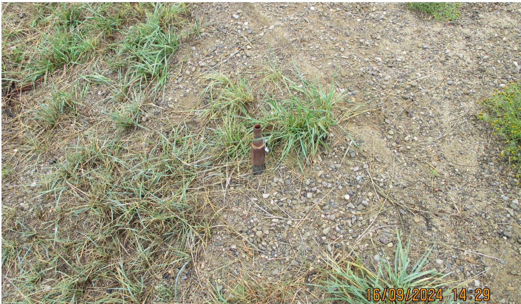
PHOTO 5: UNUSED EQUIPMENT (UNUSED UNMARKED RISER NEAR ORIG. WELLHEAD). REMOVE OR MARK UNUSED RISER PER RULE 606.
