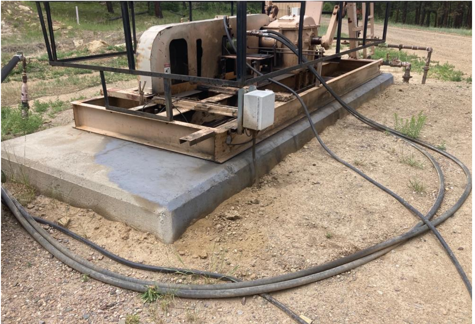
PHOTO 1: MAINTENANCE HAS BEEN PERFORMED ON ALL EQUIPMENT, THE IMPACTED SOIL HAS BEEN REMOVED AND THE CONCRETE RISER PAINTED.
