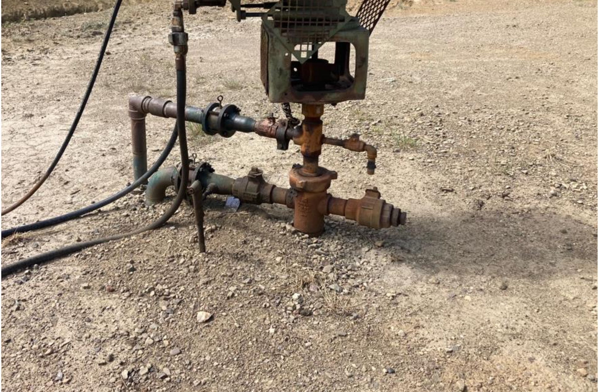
PHOTO 1: MAINTENANCE HAS BEEN PERFORMED ON ALL OPERATING EQUIPMENT, THE SOIL STAIN UNDERNEATH THE WELL HEAD HAS BEEN REMOVED AND REPLACED WITH FRESH PAD MATERIAL.
