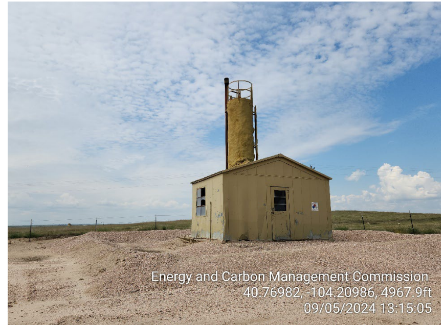
Photo 4 – Heater Treater
