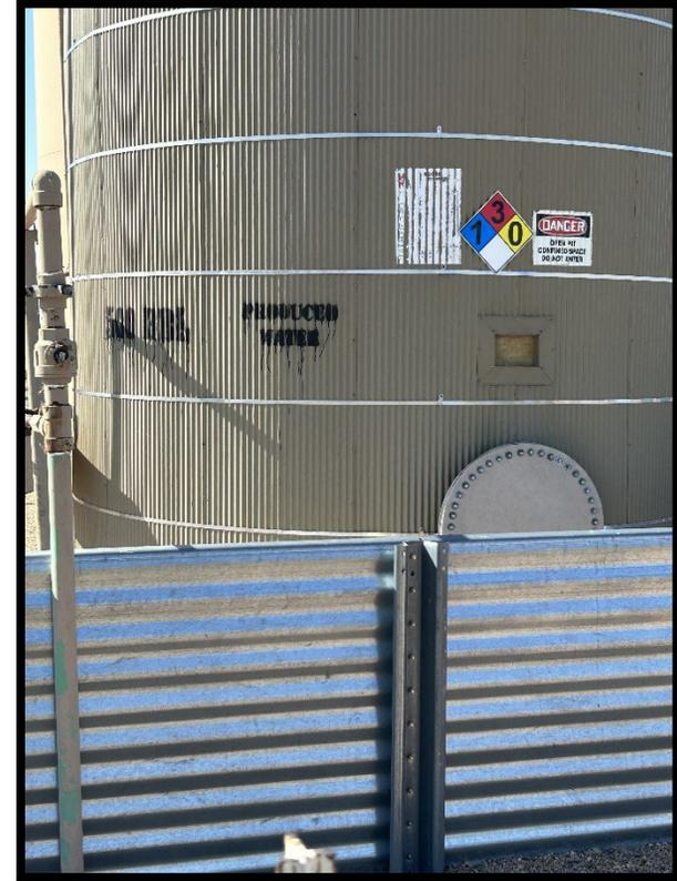
**CA:** Produced Water Tank - Missing Capacity and NFPA is fading, see photos. Comply with Rule 210.d.
