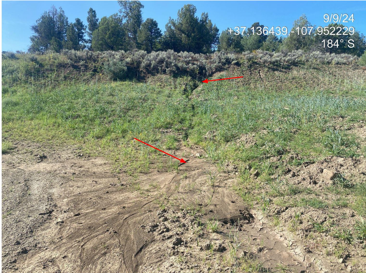
Photo 3. View of gully erosion forming in the southern portion of the contoured cut slope with evidence of sediment transport.
