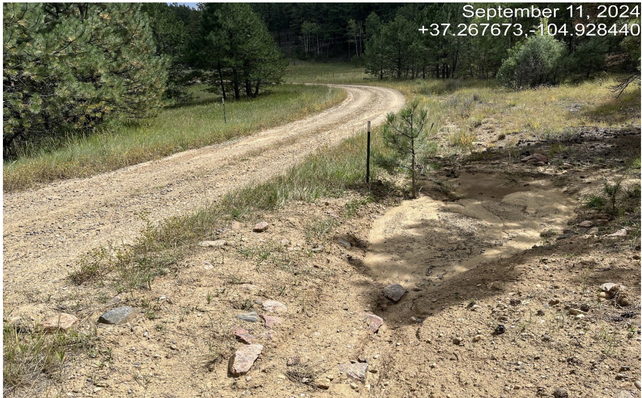
Photo 1. Facing east along the access road. This culvert is filled in with sediment.
