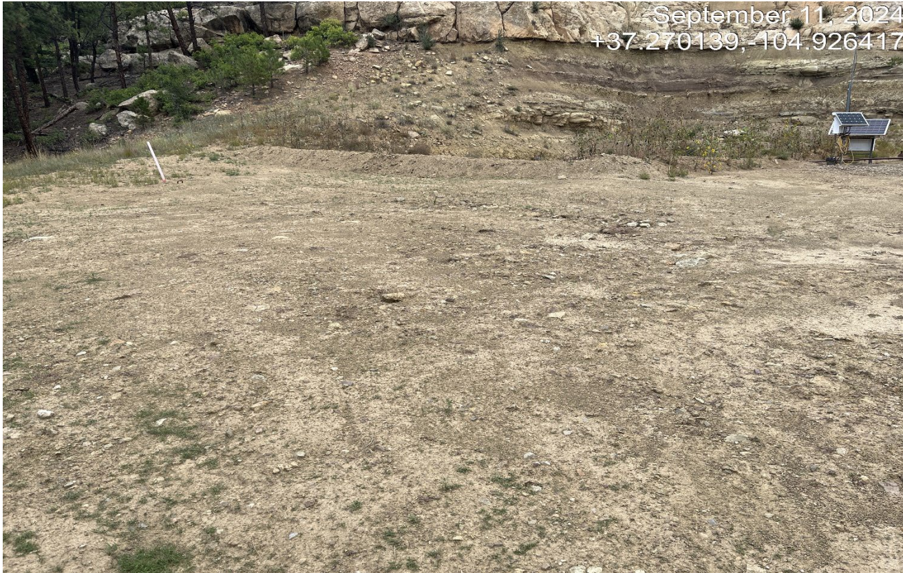
Photo 4. The pit material has been removed. It does not appear reseeding of this area has been completed and will need to be this fall.
