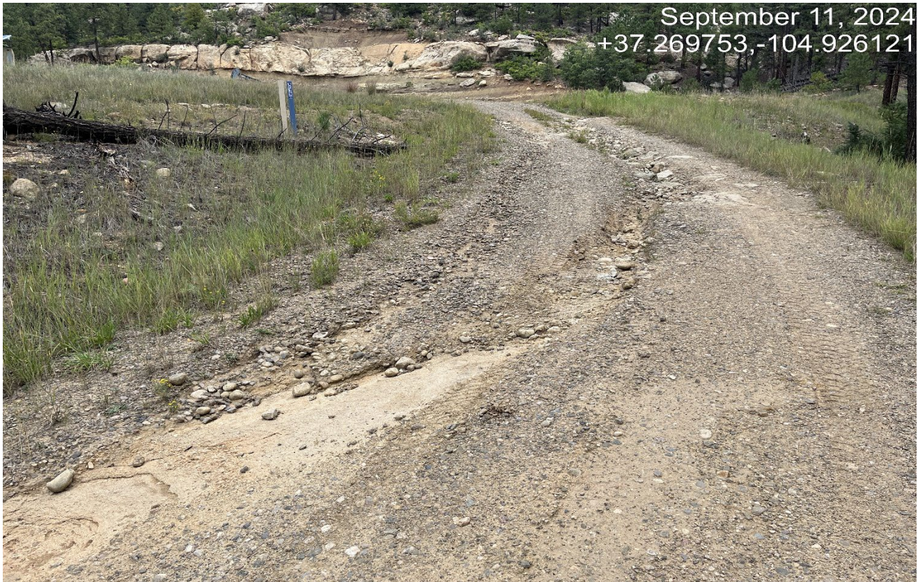
Photo 2. There is erosion of the access road at the location that needs to be repaired.
