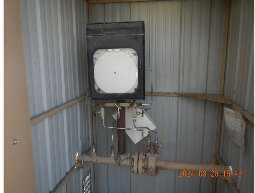
4. Gas meter inside remote meter shed.
