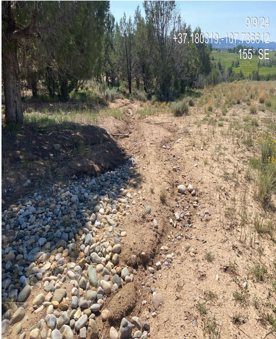
Photo 2. View of erosion observed forming in the southern interim reclamation area.
