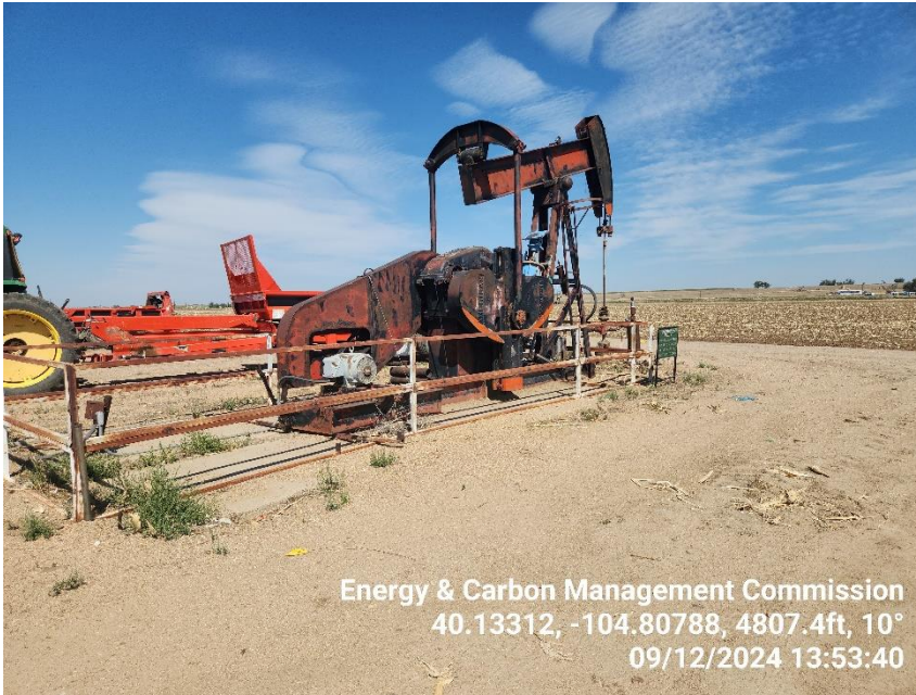
Photo 5 Pump jack prime mover
