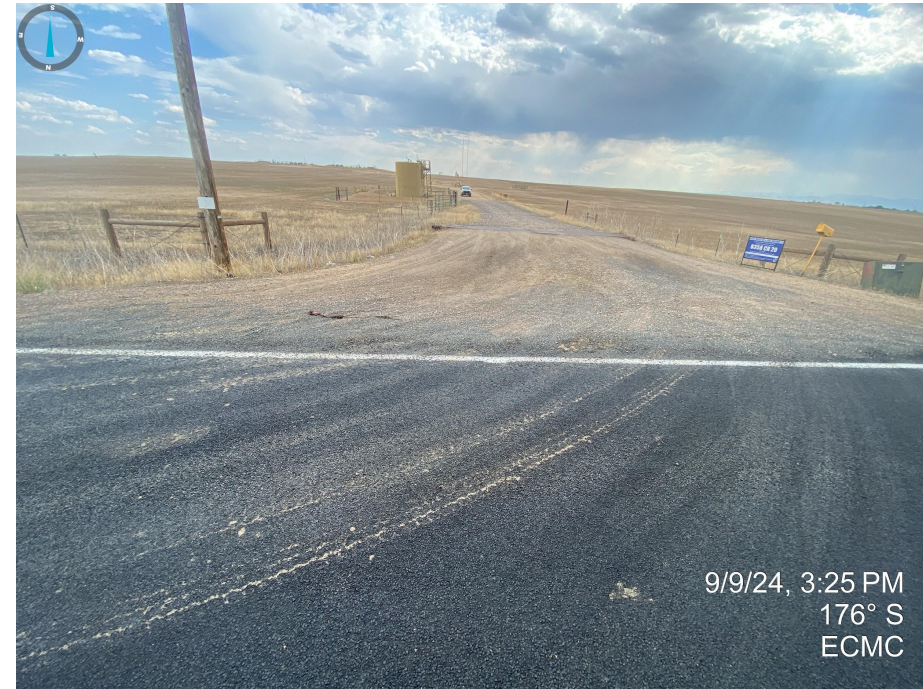
Photos 4 & 5. Photos taken from WCR 20, facing east (left photo) and south (right photo). Photos illustrate vehicle track out onto county road.
