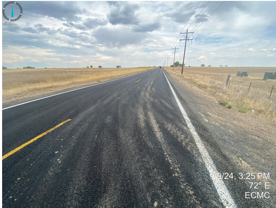
Photos 4 & 5. Photos taken from WCR 20, facing east (left photo) and south (right photo). Photos illustrate vehicle track out onto county road.
