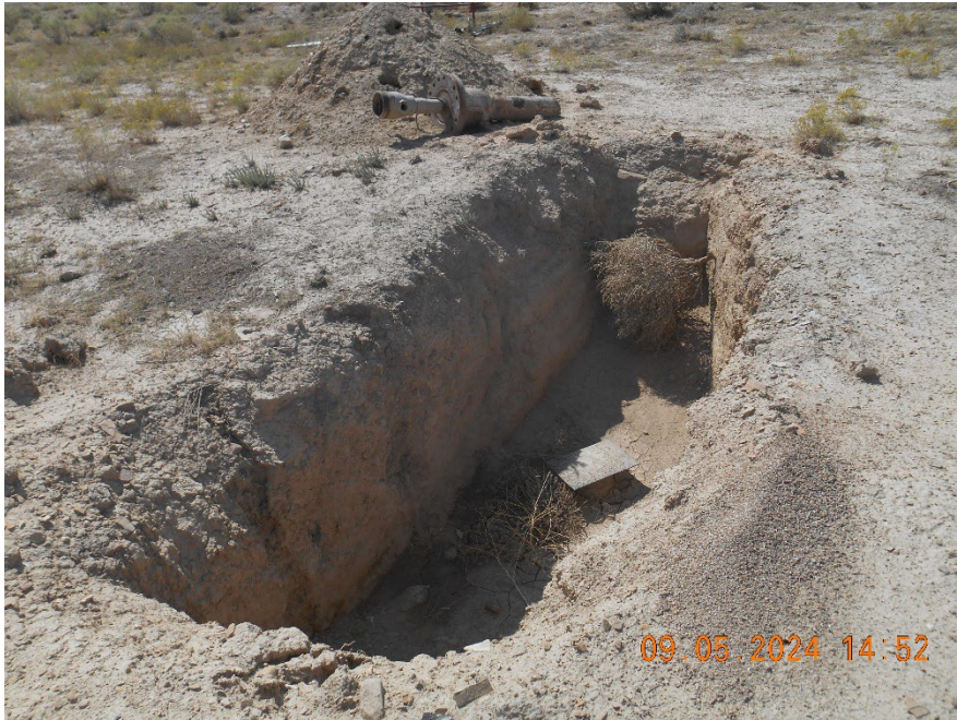
Cutoff Wellhead with welded on info plate
