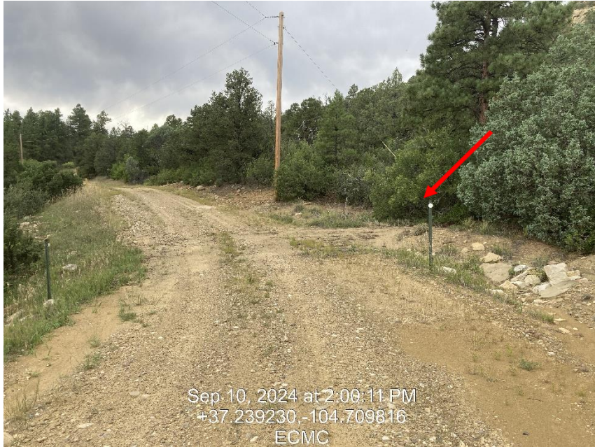
Photo 6 –Stormwater is running across access road causing erosion
