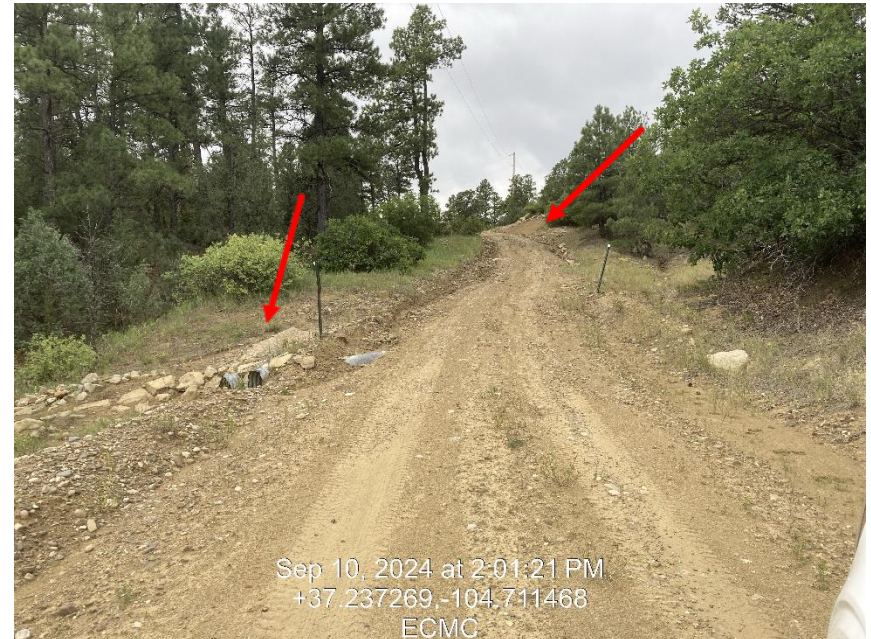
Photo 7 –Stormwater is running down the access road causing erosion
