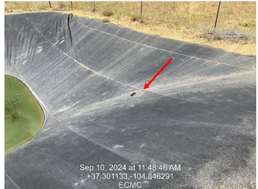
Photo 5 – Hole in pit liner
