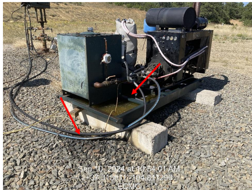
Photo 4 – Skid Pan full of oil mixed water, Stained soils observed at base
