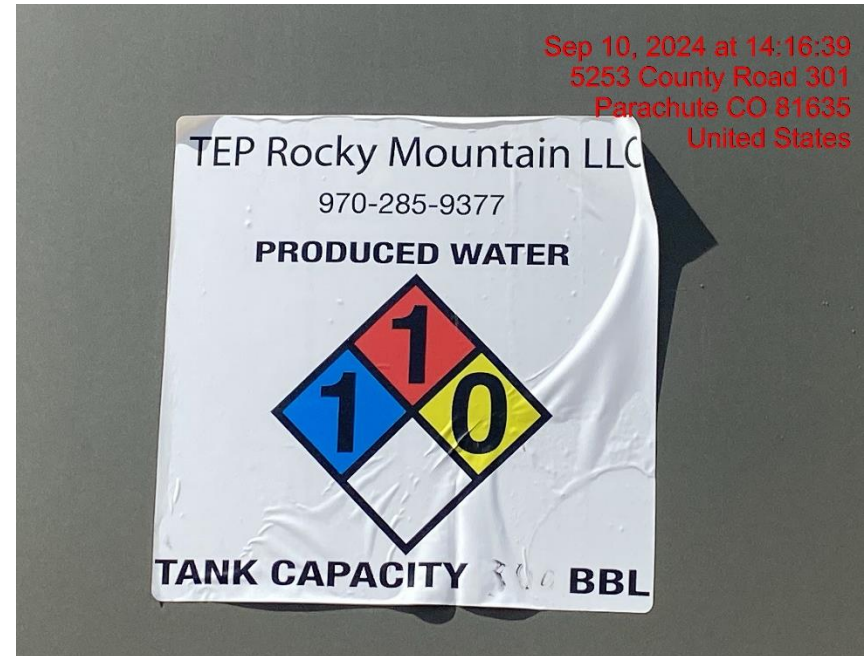
Illegible Tank Capacity on Tank Label – Photo #03351
