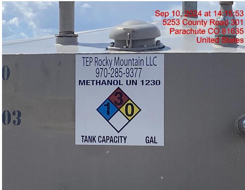
Tank Label Missing Tank Capacity – Photo #03350
