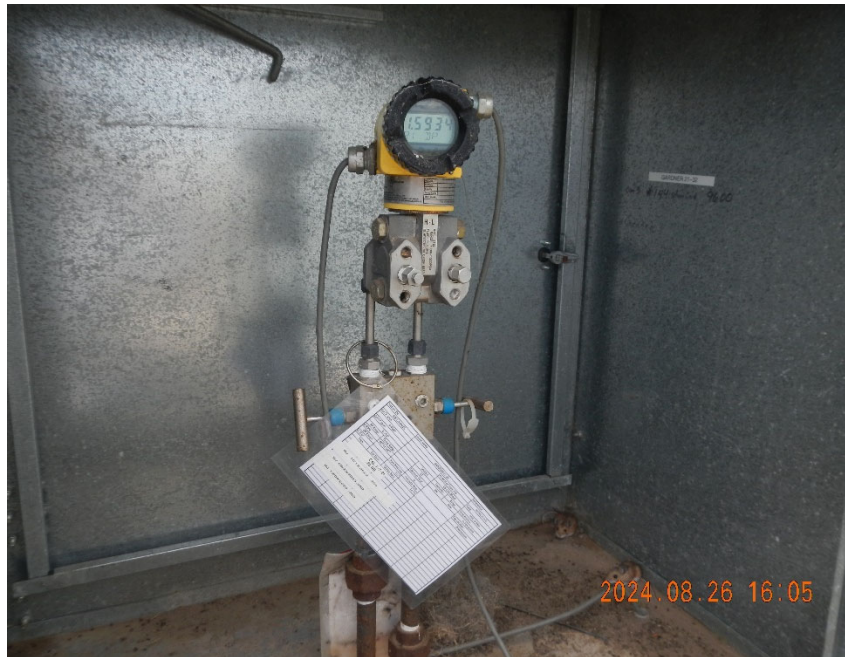
3. Gas meter inside meter box.
