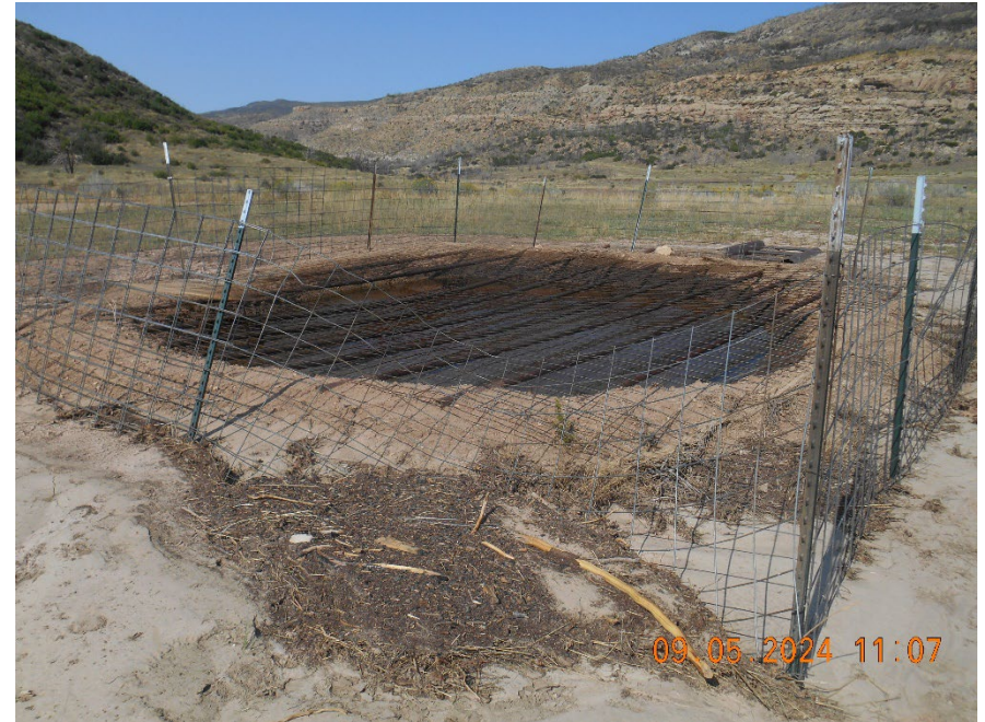
Pit with fence
