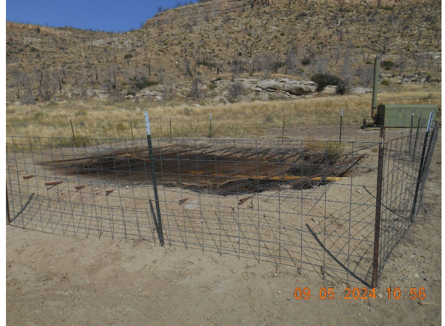
Pit with fence
