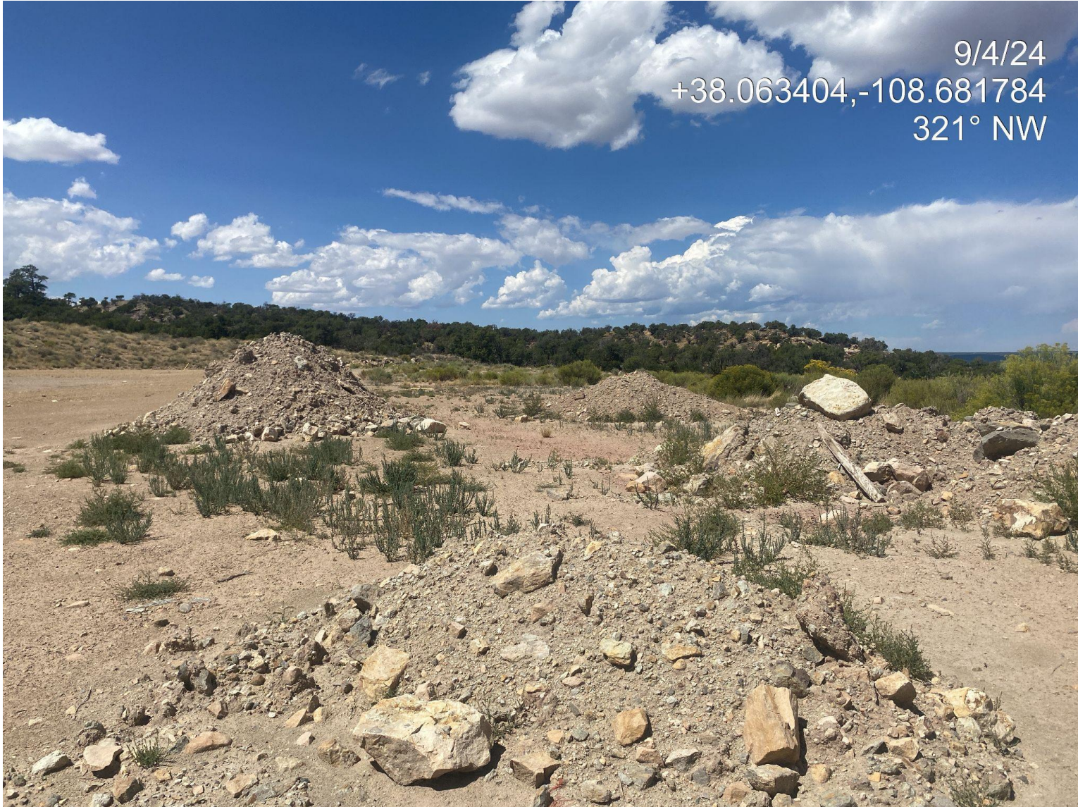
Photo 2. View of several piles of bare/loose soils stored around the location with no erosion/sediment transport BMPs in place.
