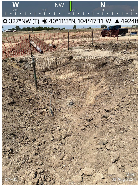
Wellhead Excavation
