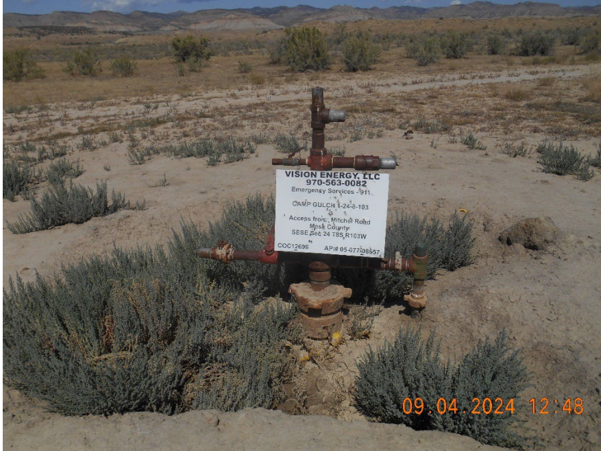
Wellhead with sign
