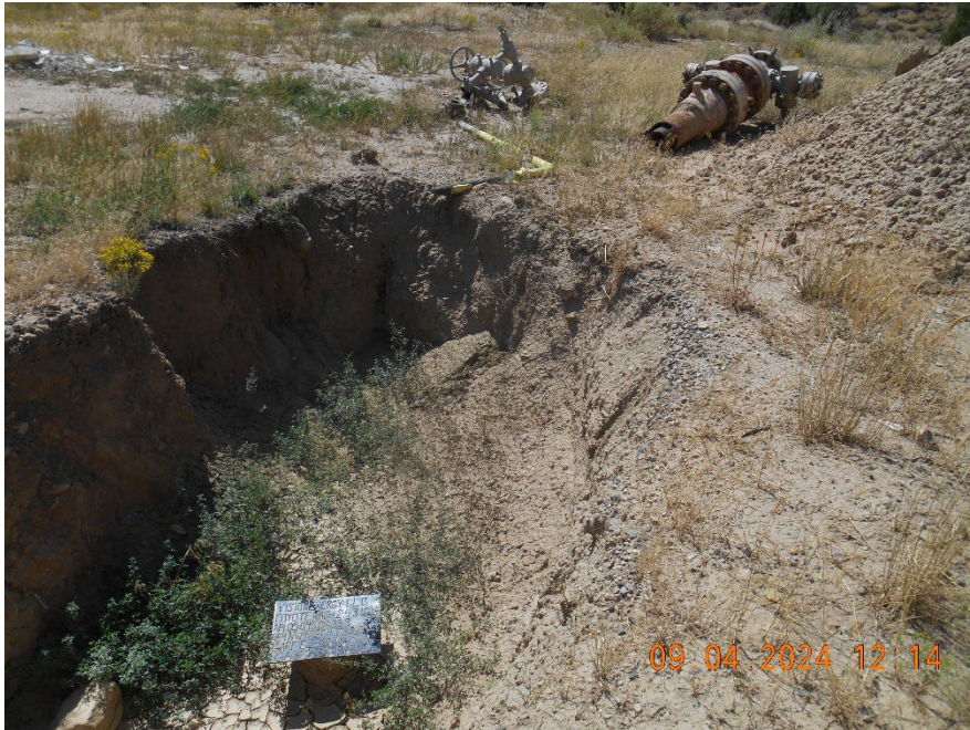
Cutoff Wellhead with ID plate welded on.
