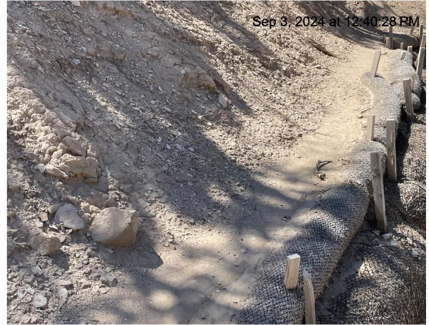
Photo # 7798 Large amount of sediment building up at waddles on slopes around tank battery/may need maintenance in near future
