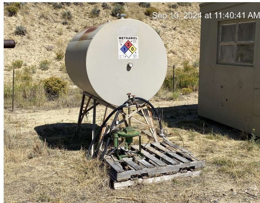
No secondary containment
