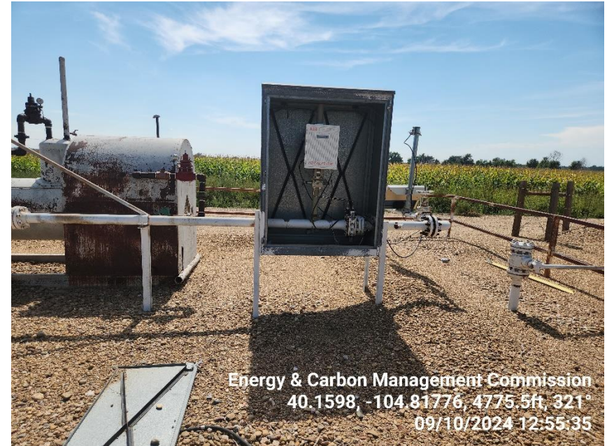
Photo 8 Gas Meter Run.
