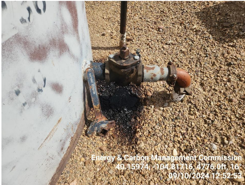
Photo 5 Stained soil by the TB valve.
