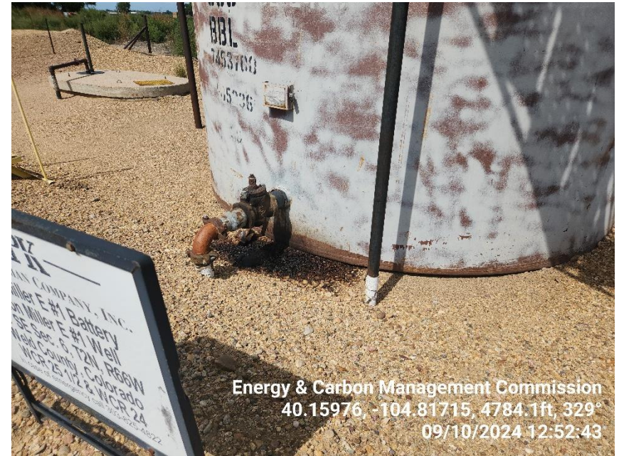
Photo 4 Stained soil by the TB valve.
