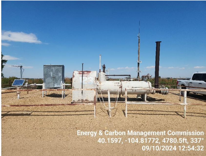
Photo 7 Horizontal heated separator, Gas Meter Run & telemetry.
