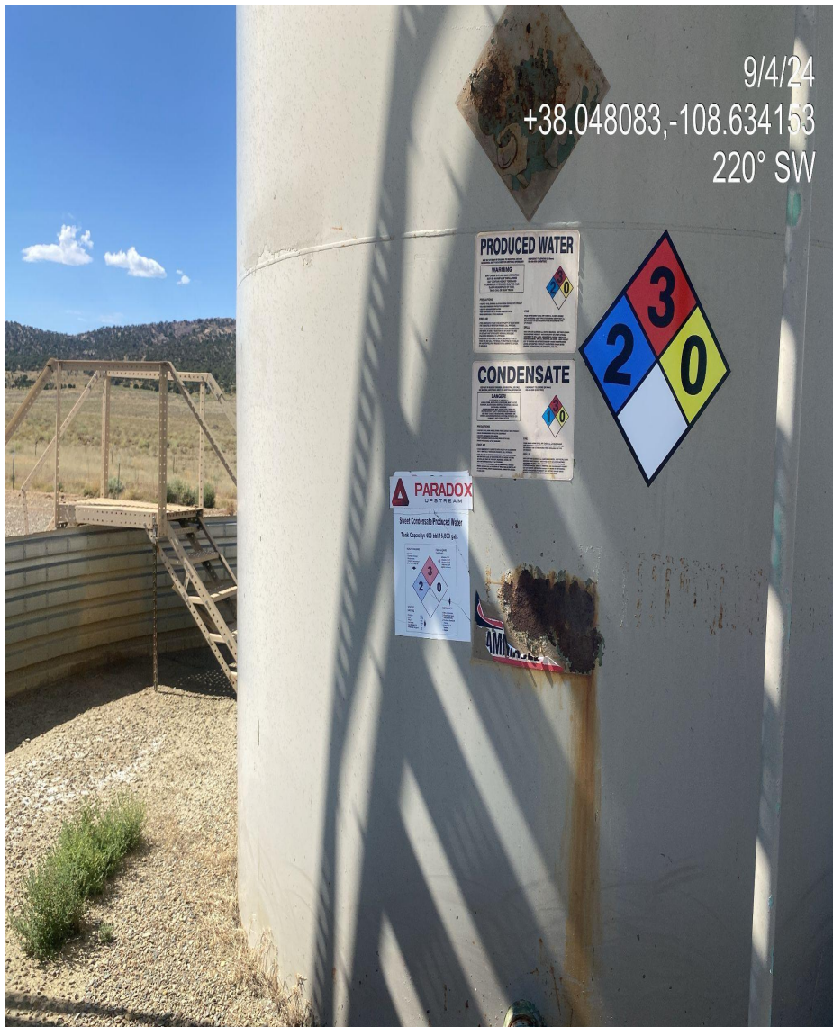
Photo 4. Signs at produced water tanks need to be updated. Per rule 605.g buying operator has 60 days from approved form 9 date to replace or update signs on location.
