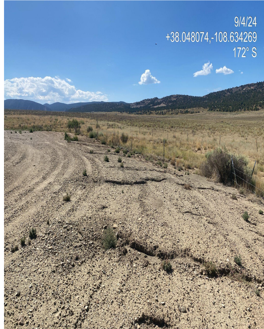
Photo 3. Several erosional channels observed in the southern portion of the disturbance. Stabilization/stormwater BMPs needed in this area.
