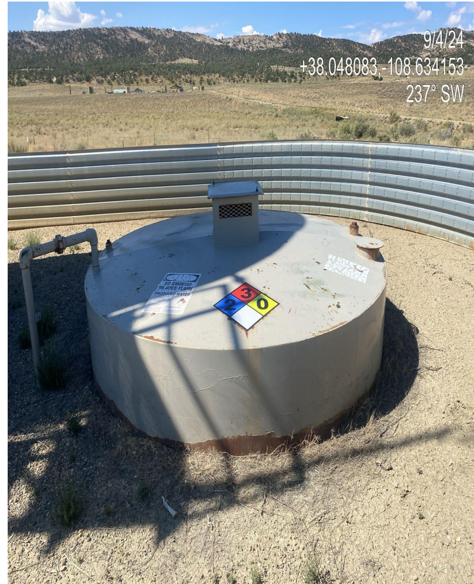
Photo 4. Signs at produced water tanks need to be updated. Per rule 605.g buying operator has 60 days from approved form 9 date to replace or update signs on location.
