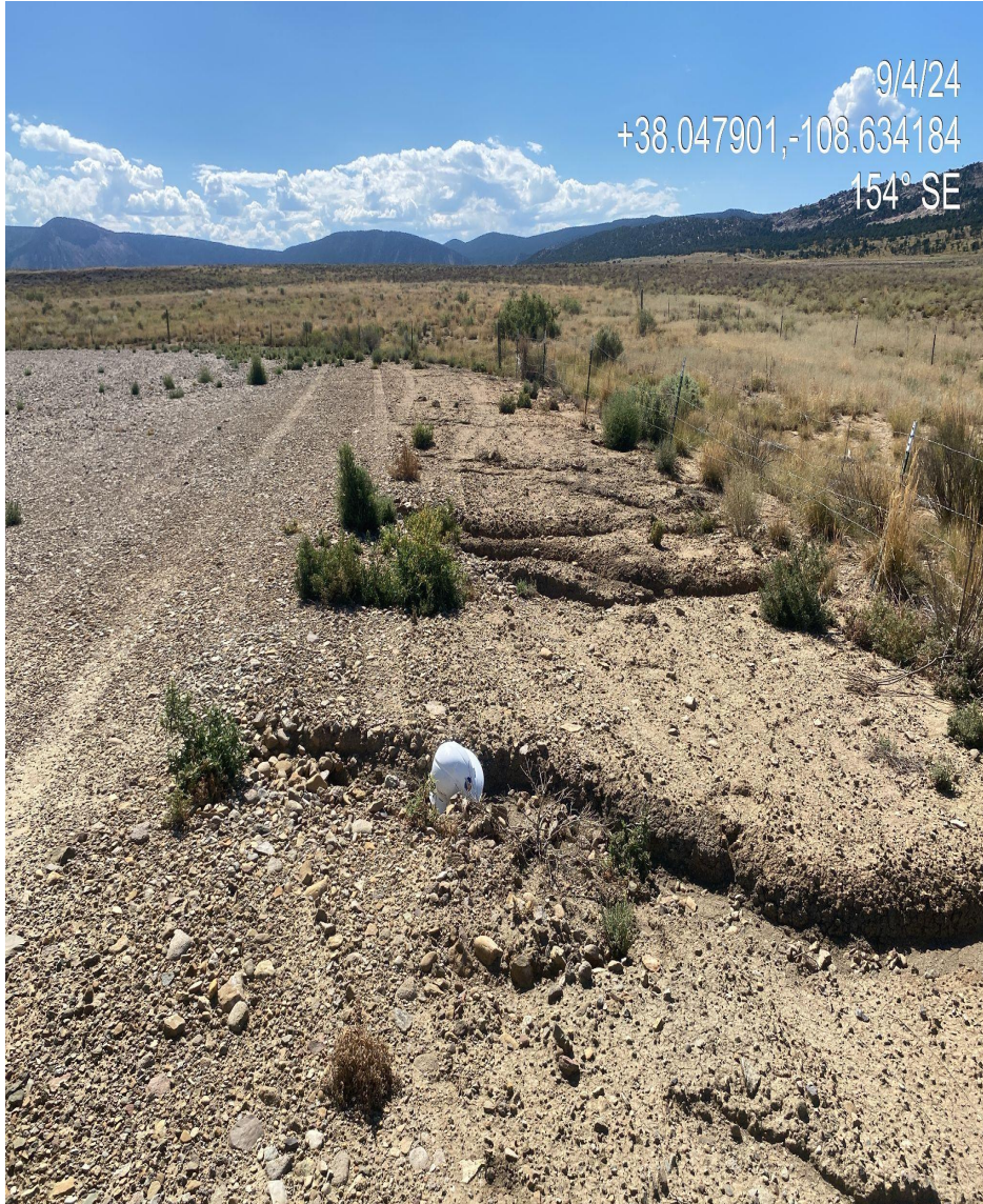
Photo 3. Several erosional channels observed in the southern portion of the disturbance. Stabilization/stormwater BMPs needed in this area.
