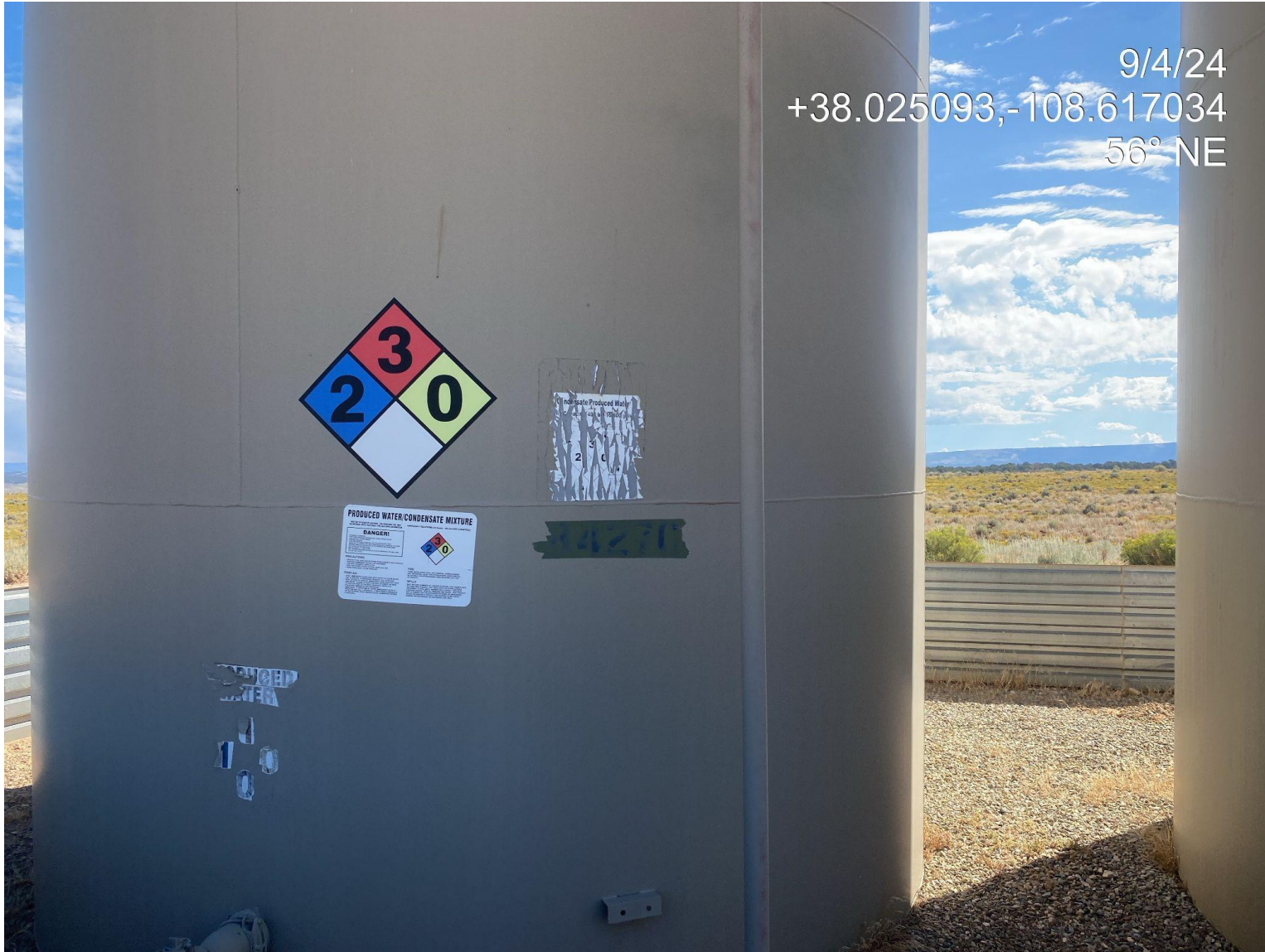
Photo 2. Signs at produced water tanks need to be updated. Per rule 605.g buying operator has 60 days from approved form 9 date to replace or update signs on location.
