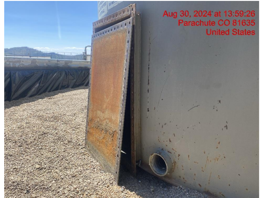
Unsecured Equipment/Wildlife Entry Hazard – Photo #03290
