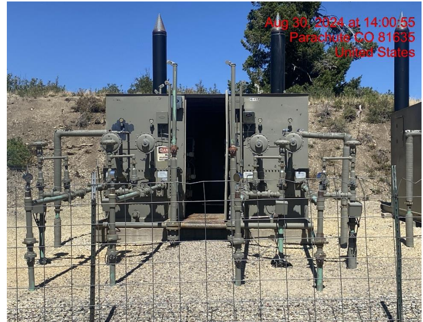
Unsecured Equipment/Wildlife Entry Hazard – Photo #03295
