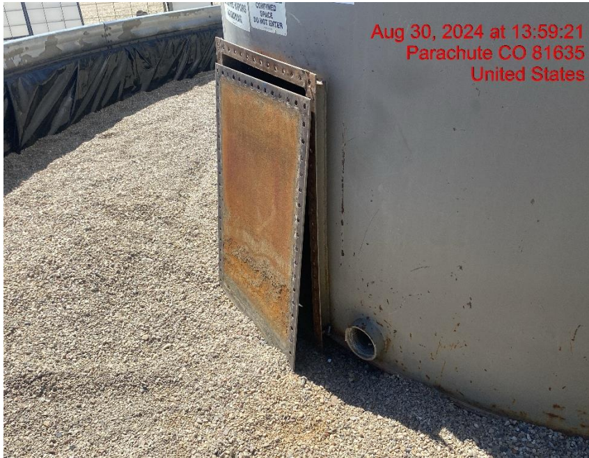
Unsecured Equipment/Wildlife Entry Hazard – Photo #03289
