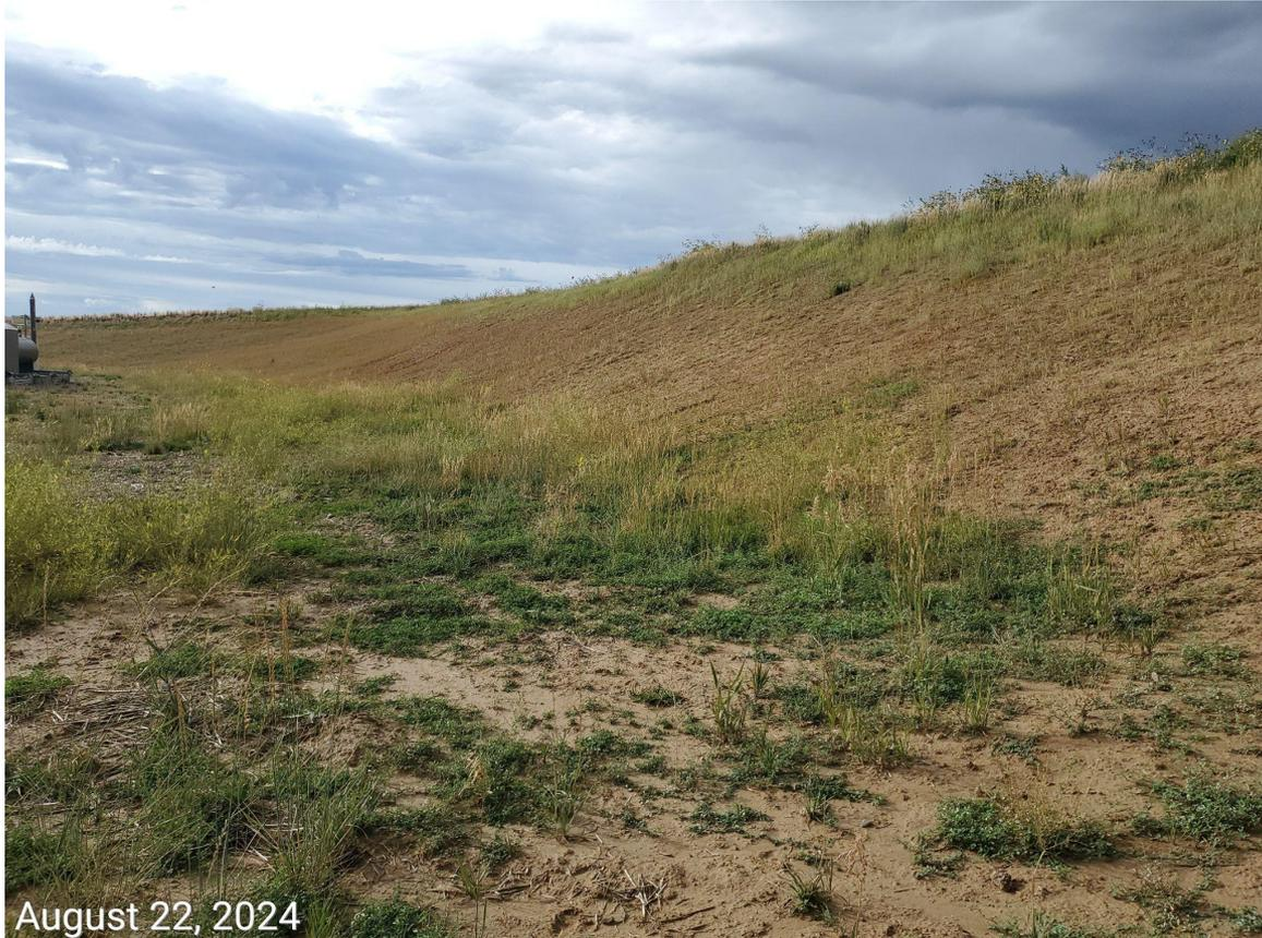
**Photo 11:** Photo taken from the west end of the Location facing southeast. Photo shows cut slopes have been recontoured. Vegetation establishing on the slopes are predominantly undesirable plant species.
