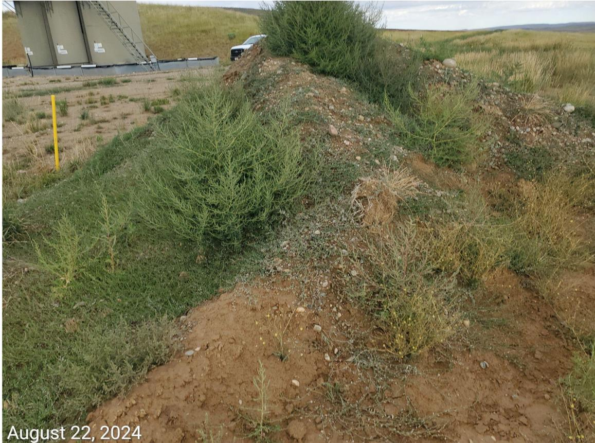
**Photo 5:** Photo taken from the northeast end of the working pad surface. Photo shows stockpile of material stored on Location. Photo also shows that BMPs to protect the stockpile from wind/water erosion, BMPs to minimize sediment transport, and BMPs to protect stockpile from weed establishment are missing or insufficient. BMPs required pursuant to Rule 1002.c and 1002.f, or, If materials are not necessary, materials require removal.
