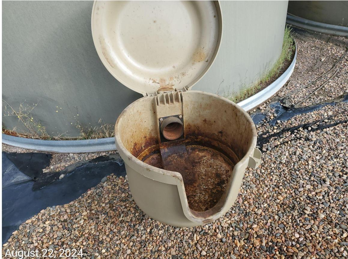
**Photo 8:** Photo taken from the tank battery facility on the north end of the Location. Photo shows line at tank has not been capped or plugged.
