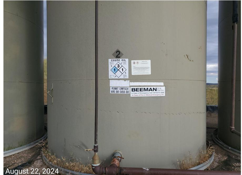
**Photo 7:** Photo taken from the tank battery facility on the north end of the Location, facing north. Photos examples showing information pursuant to Rule 605.h (NFPA Label, Capacity information) has not been posted.
