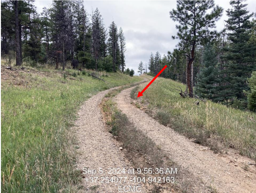
Photo 7 – Stormwater is running down the center of the access road causing riling.
