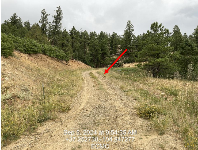
Photo 5 – Stormwater is running down the center of the access road causing riling.
