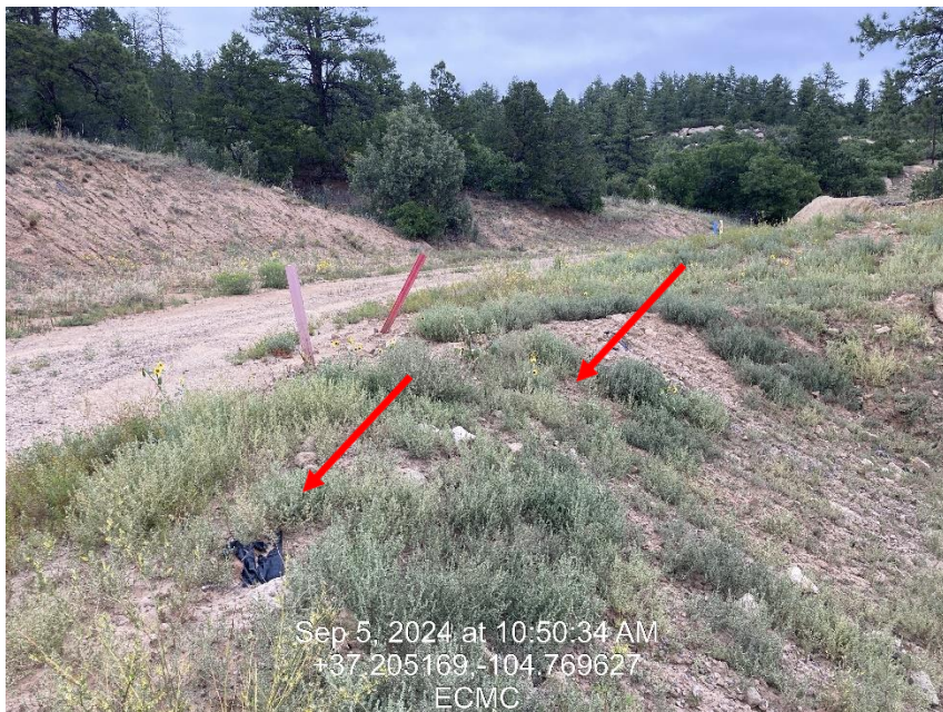
Photo 7 – Pieces of pit liner material on west edge of pit
