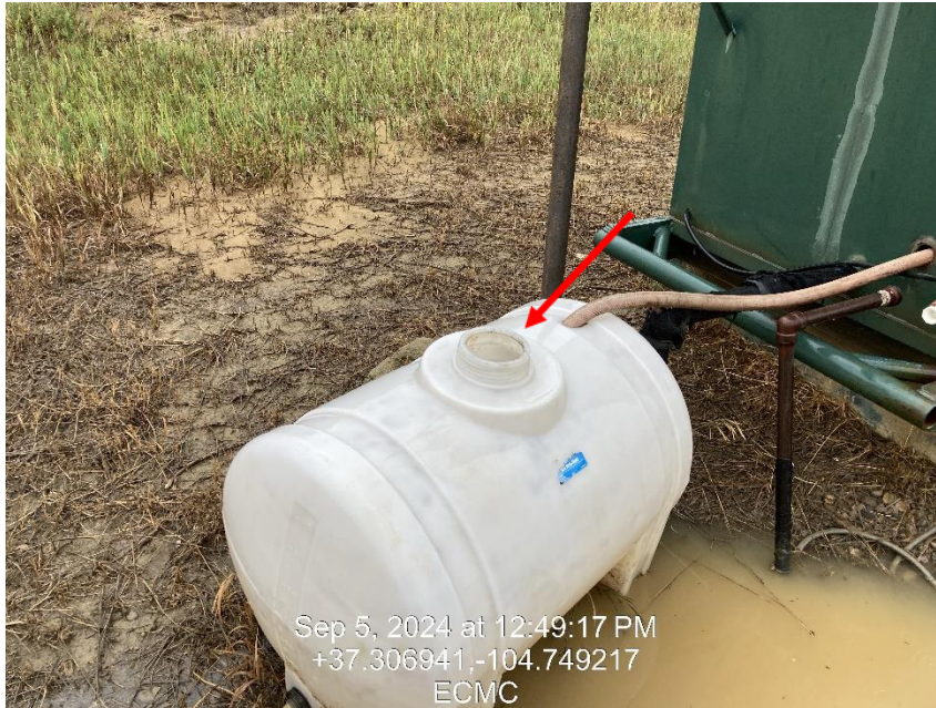
Photo 3 – Tank at meter house missing cap.
